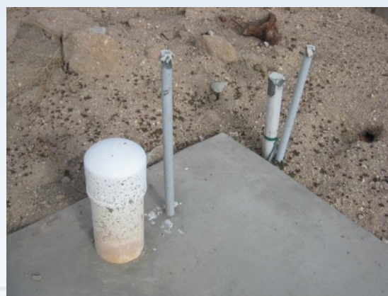
Stub outs for electrical and water conduits
